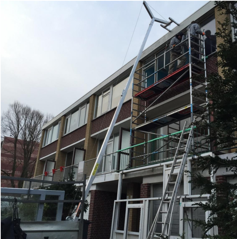
The Knight model xL over the Scaffolding, 5.5 to 10 meter 250 kg.
